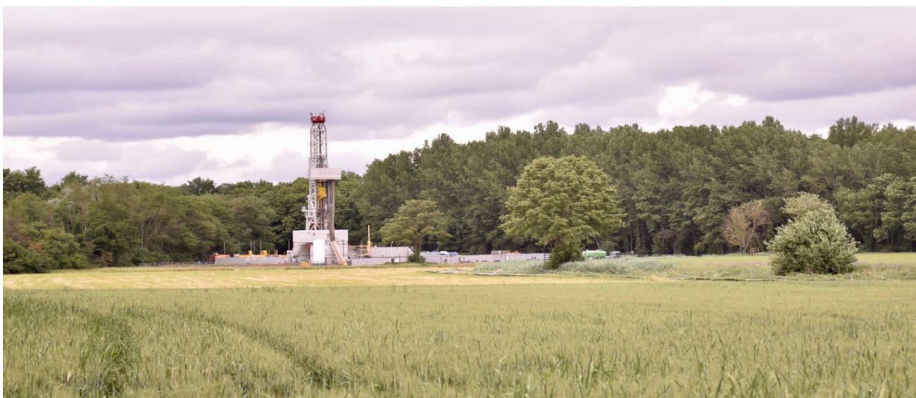
• WELL STEIG 1 OF RHEIN PETROLEUM
