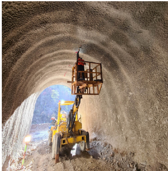
“MONTY B PORTAL” ACCESS SHAFT, SANGDONG MINE, SOUTH KOREA
