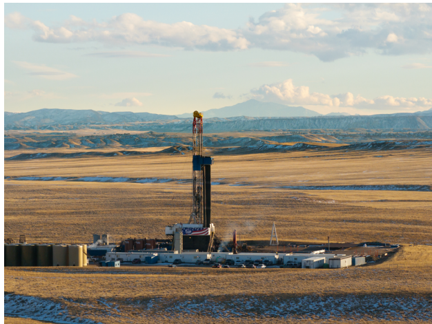
Drilling by Bright Rock Energy
