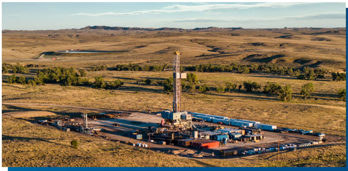
1876 RESOURCES WELL ON THE NETZ PAD, WYOMING
