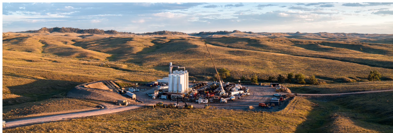
COMPLETION OF WELLS, WYOMING
