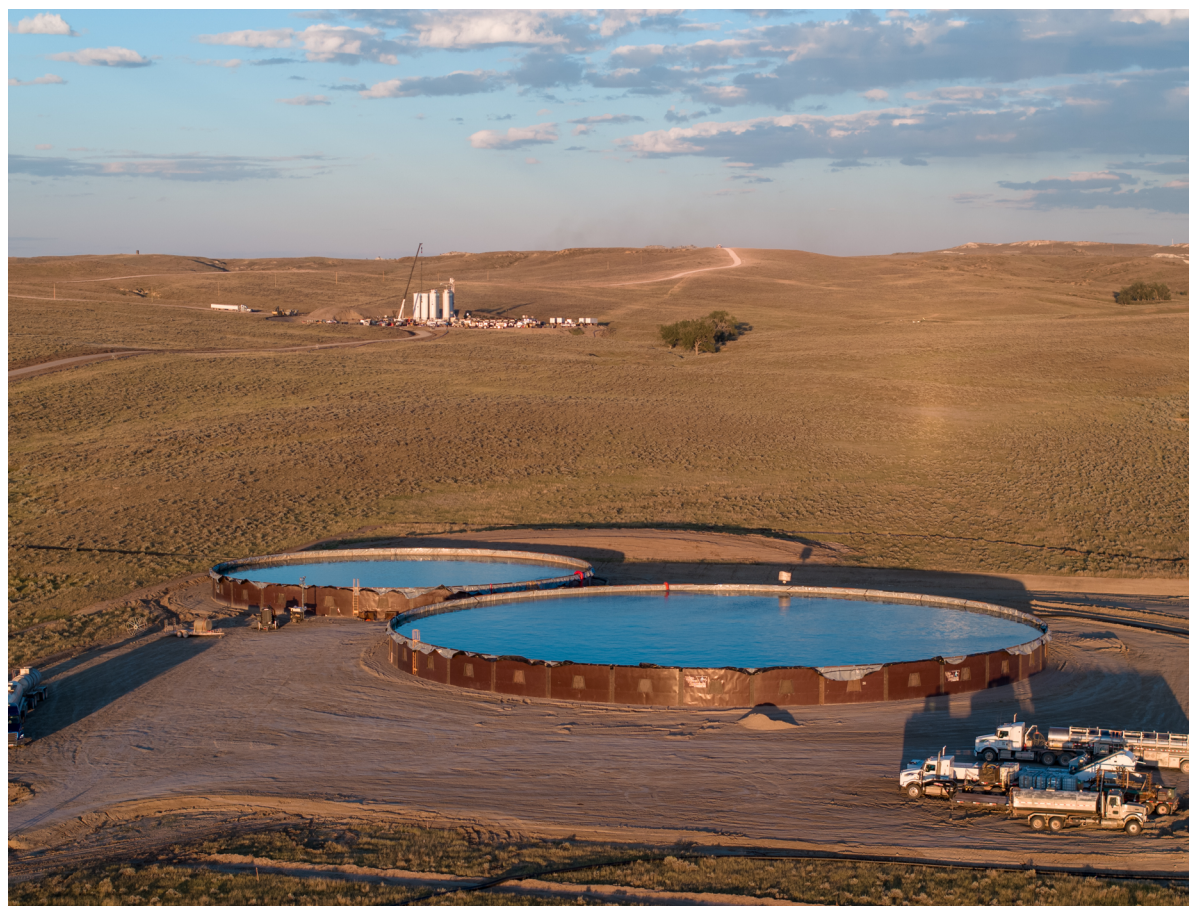
WATER STORAGE FOR COMPLETION, WYOMING.
